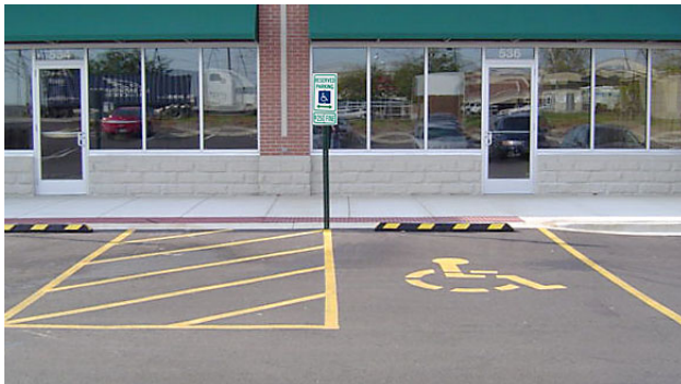
Above: Example of an accessible parking space that complies with Illinois law.
